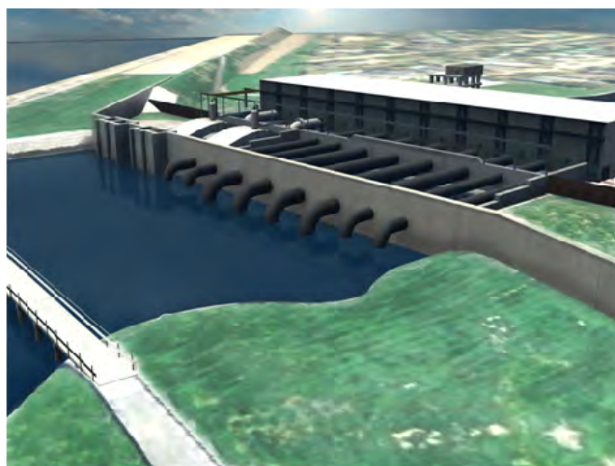
Pump Station with Fronting Protection
